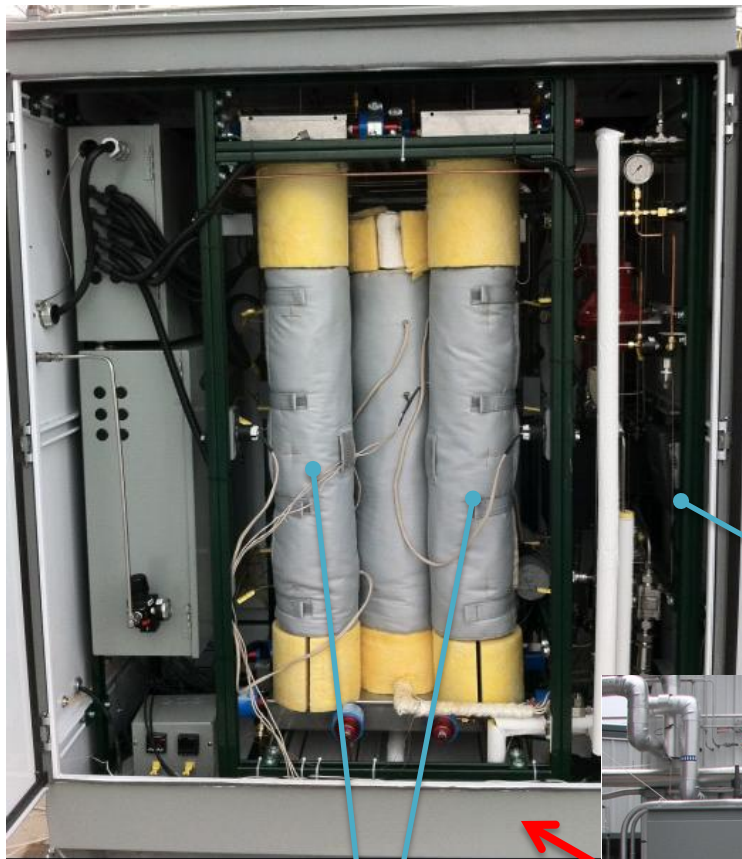
Cabinet #2- CO 2 Removal
